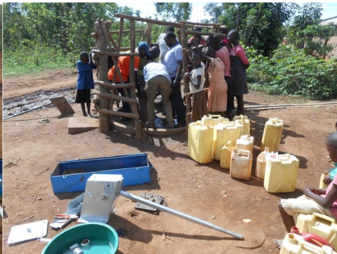
Fixing in new system in the broken borehole
