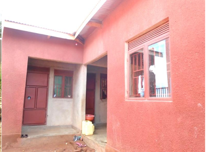
On left Staff houses after plastered on right After fixing in glasses with redoxide wall color
