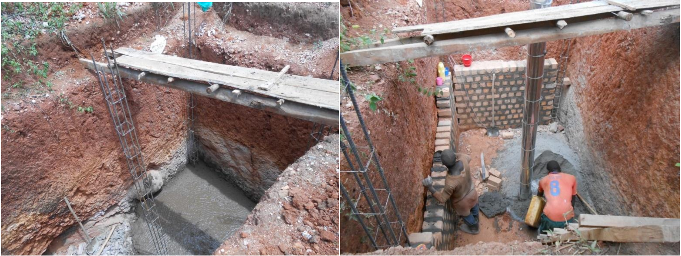
From left to right the pit basement with concrete and Building brick walls of the pit
