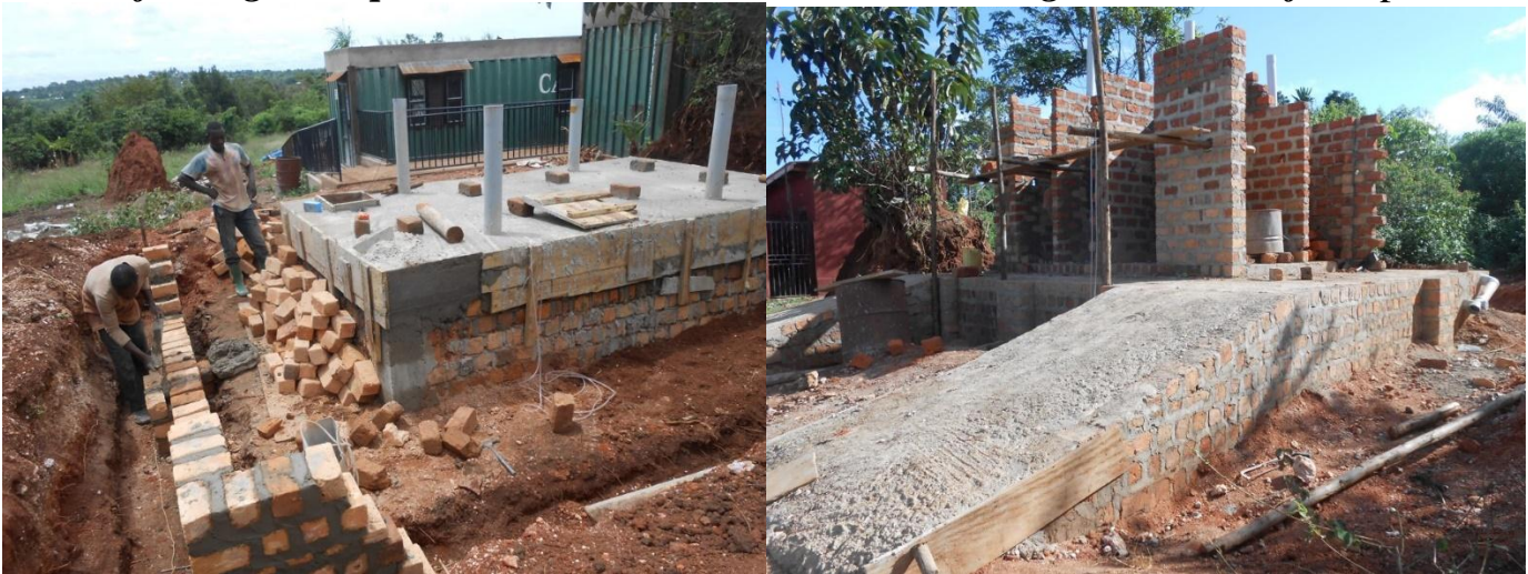
Finishing the slab and the progress work of the super structure wall for pit latrine.
