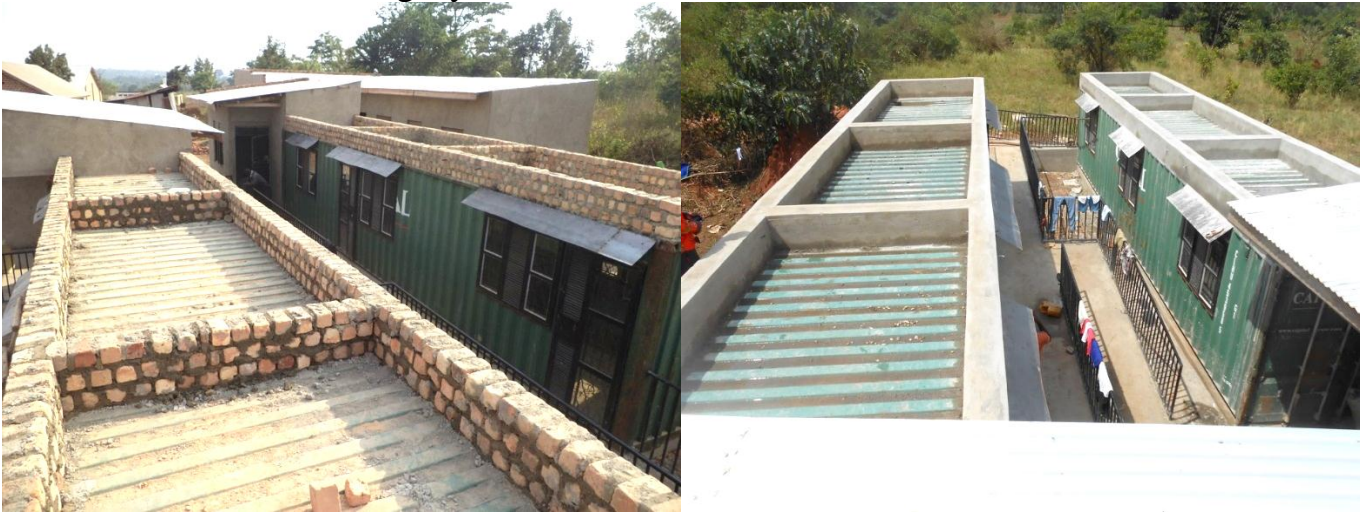
Built brick boxes, on right after doing finishing works on built roof brick container boxes
