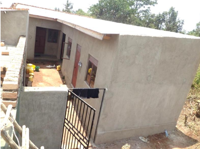
On left Staff houses after plastered on right After fixing in glasses with redoxide wall color
